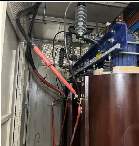
Cast Rasin Transformer
